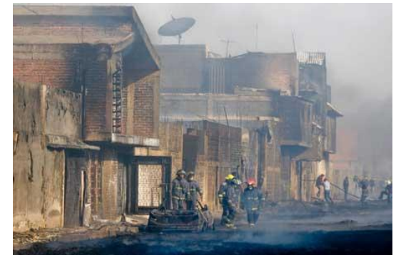
Pipeline explosion in Puebla, Mexico 2010
